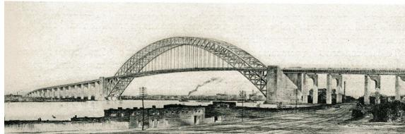
Figure 5: Original Design of the Bayonne Bridge. *This is a sketch of the original design of the Bayonne Bridge with its towers (courtesy of the Port Authority of New York and New Jersey, Source: “First Progress Report on Kill van Kull Bridge” [Ammann 1930a]).*
